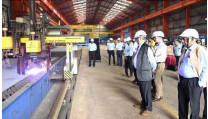
Steel cutting of 2 nos. of 3800 tonnes dry cargo vessel being built for M/s. Wilson Ship owning AS, Norway was held at UCSSL on 04 th December, 2023
