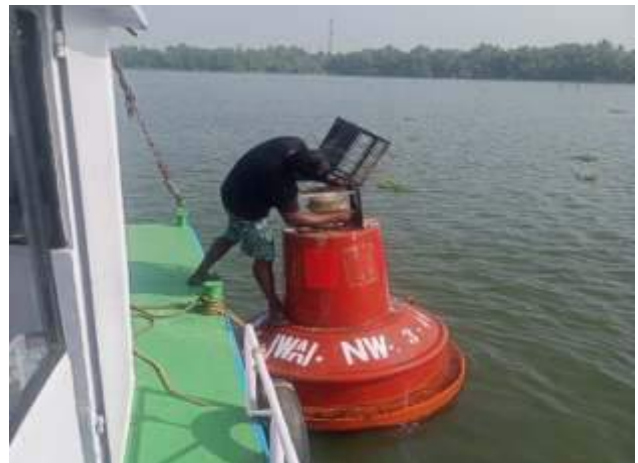
Solar Powered FRP Buoy installed in NW-3 on 05th October 2023
