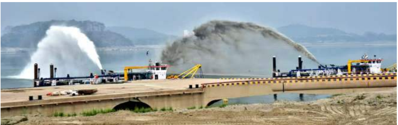
Maintenance dredging in NW-3
