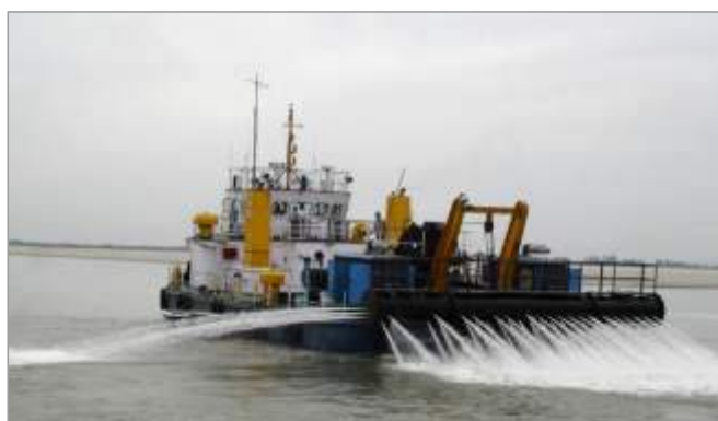
Hydraulic Surface Dredger deployed in NW-2
