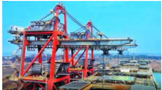
Mechanised Coal handling at berth No.16 (PPP)
