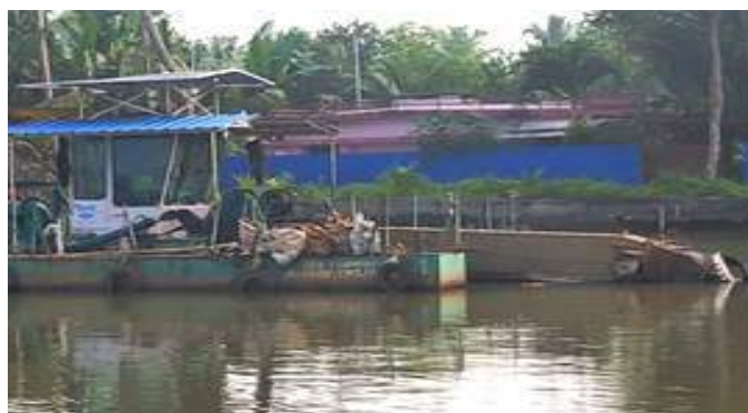
Maintenance dredging with Department Dredger “CSD Champakkara” in NW-3
