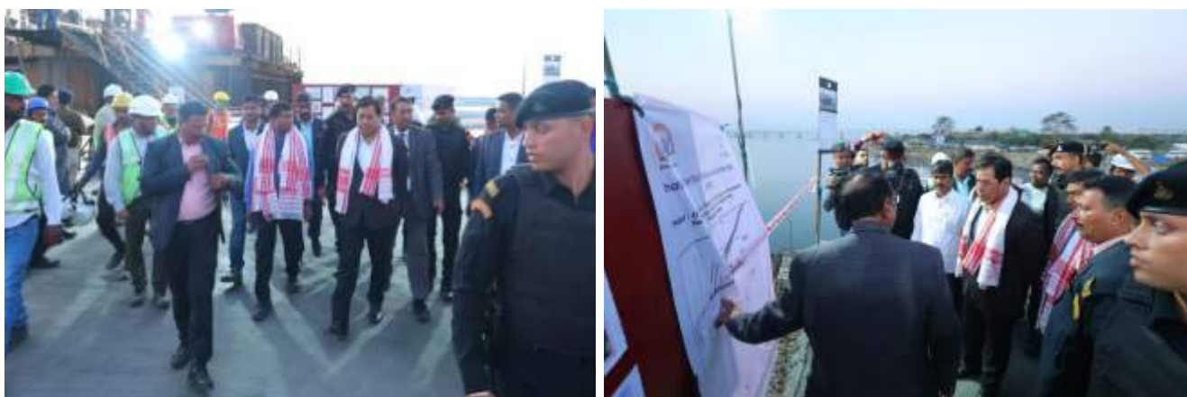
Hon'ble Minister PS&W inspected the project site of Tourist cum Cargo Jetty at Bogibeel, Assam on 25th December, 2023
