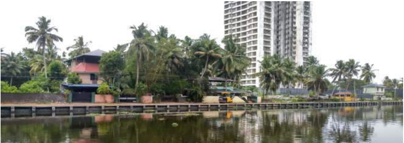
Pile and slab type bank protection work in Cahmpakkara Canal
