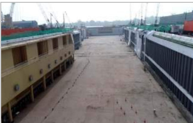
Dock floor of New Dry-dock at Cochin Shipyard Limited
