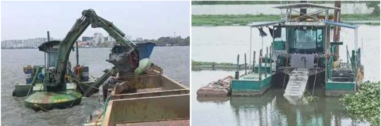
Maintenance dredging in NW-3
