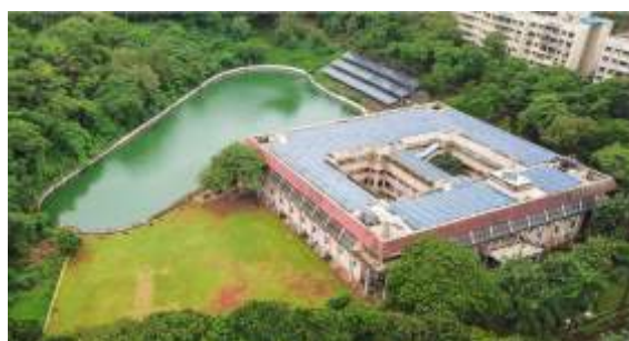
Maritime Training Institute, Powai Ariel View
