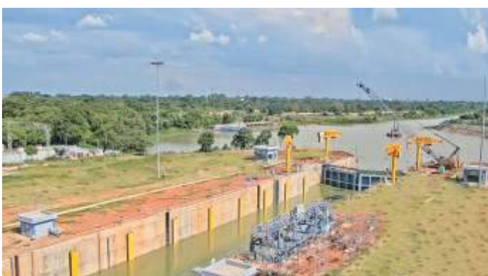
New Navigational Lock Gate, Farakka, West Bengal
