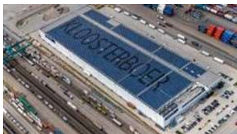
Figure 17 Rooftop Solar Panels in Port of Rotterdam
