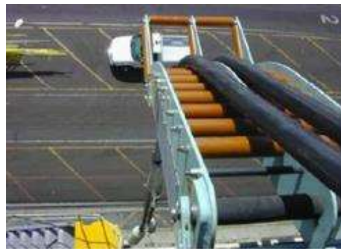
Figure 8 Cables for connection
